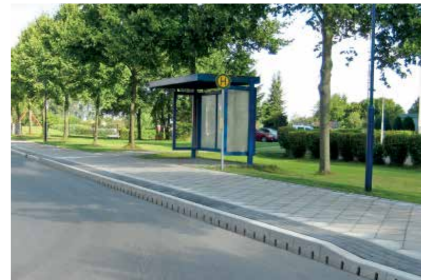
ACO DRAIN® KerbDrain system is used at a bus stop: Passengers enter the bus unobstructedly with the aid of the 18 cm high kerb.
