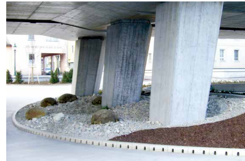
Kerbstone and drain in one, ACO DRAIN® KerbDrain
