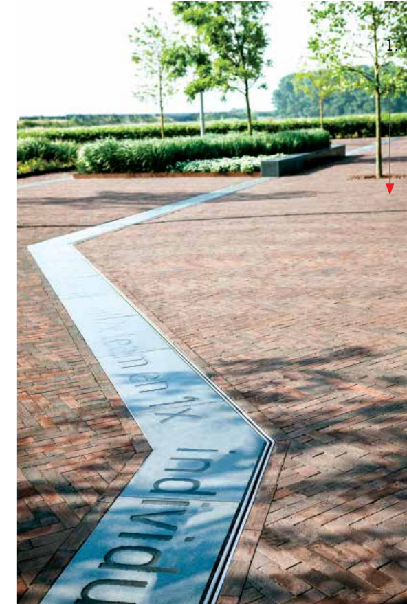
The plastic body of the ACO XtraDrain channel with a slotted frame
